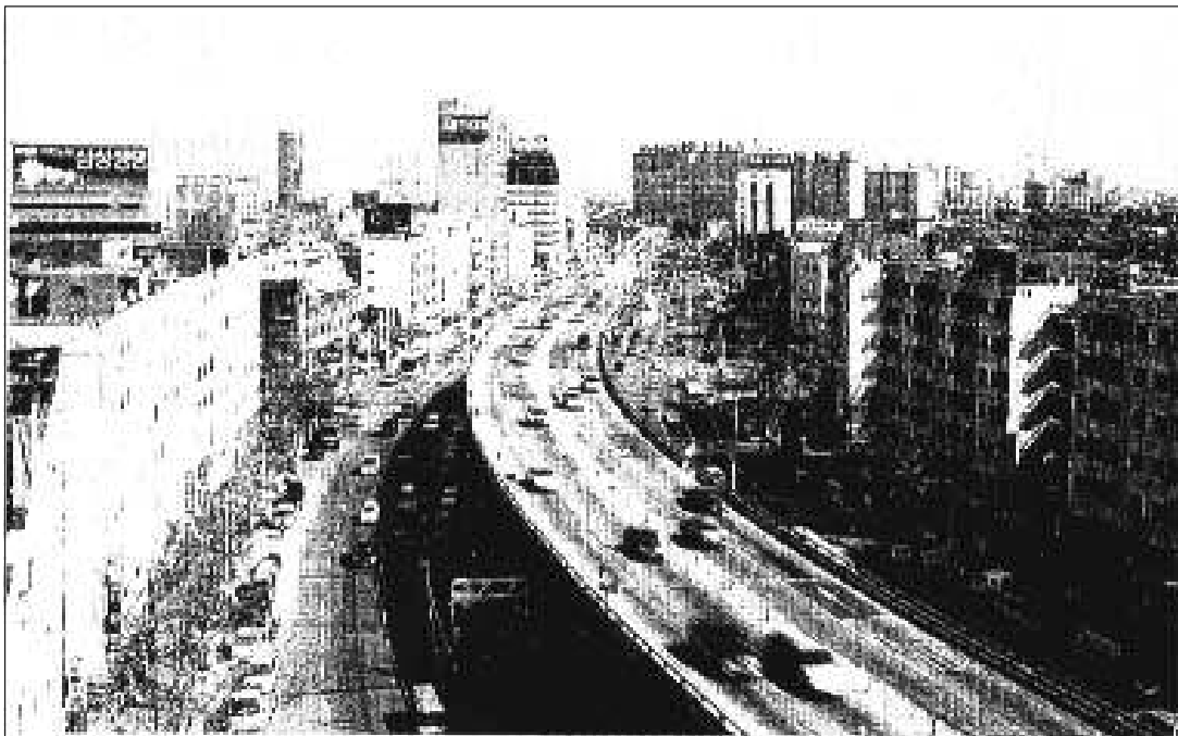
Fig. 1.12. Elevated Expressway before demolition
