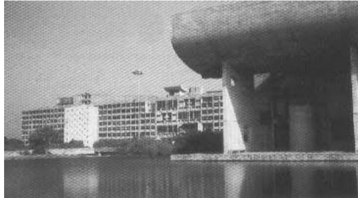
Fig.1.21: Le Corbusier's Chandigarh, the Secretariat and Legislative Assembly, constructed from 1956 to 1970, became the testing ground for many of the architect's ideas on how to design for the combination of extreme summer heat and cool winters. Huge brise-soleils dominate the assembly building. The device for creating shade had come of age. Chandigarh as the administrative capital comprised a series of buildings: the Secretariat, the Assembly, the Governor's Palace, and the High Court. In developing his design for the complex, Le Corbusier drew on the skills of traditional Mughal building, notably Fatehpur Sikri.
