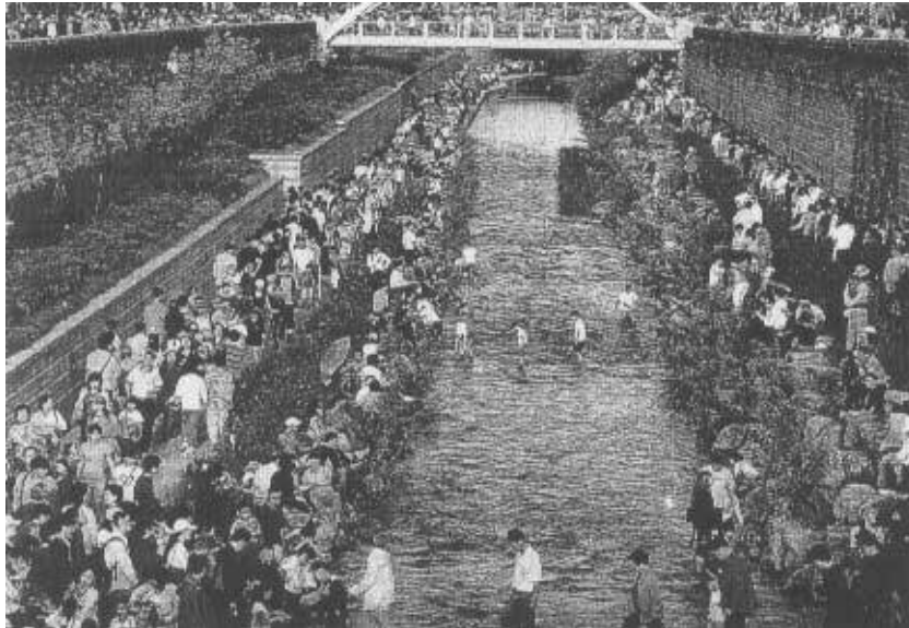
Fig. 1.13 Recovery of river by dismantling elevated expressway in Seoul, Korea
